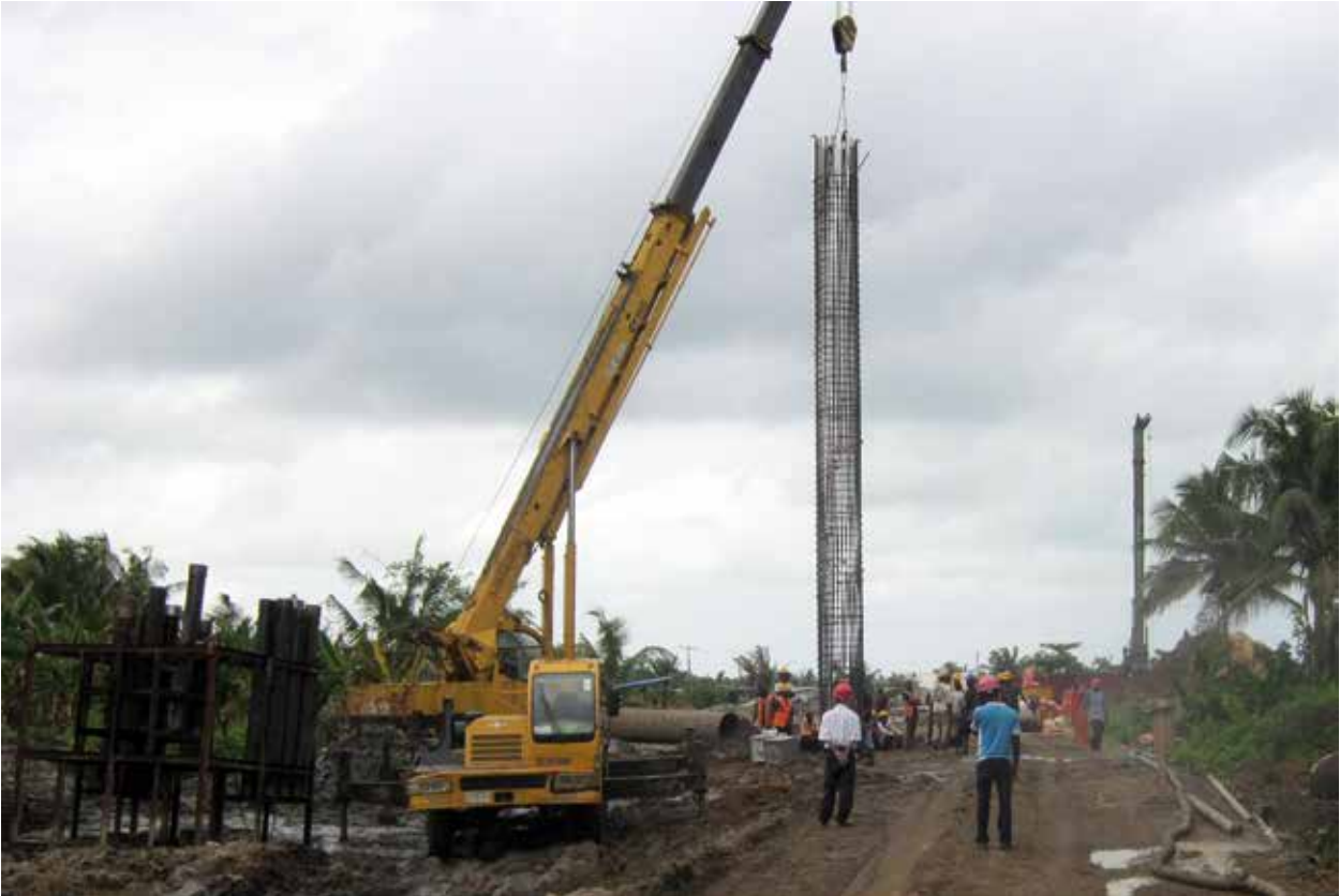
Construction of Aradagun-Iworo-Ajido (Phase 1), Bridge Only (Section 1) in Badagry Local Government Area Client: CCECC NIGERIA LTD Bored piles
