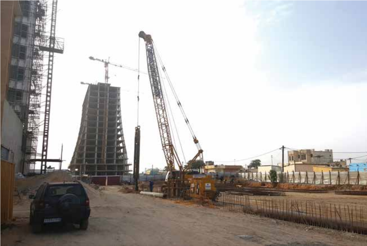
Residential Development, Nouakchott, Mauritania Client: SMID (WAFA GROUP) Diaphragm Walls and Anchors
