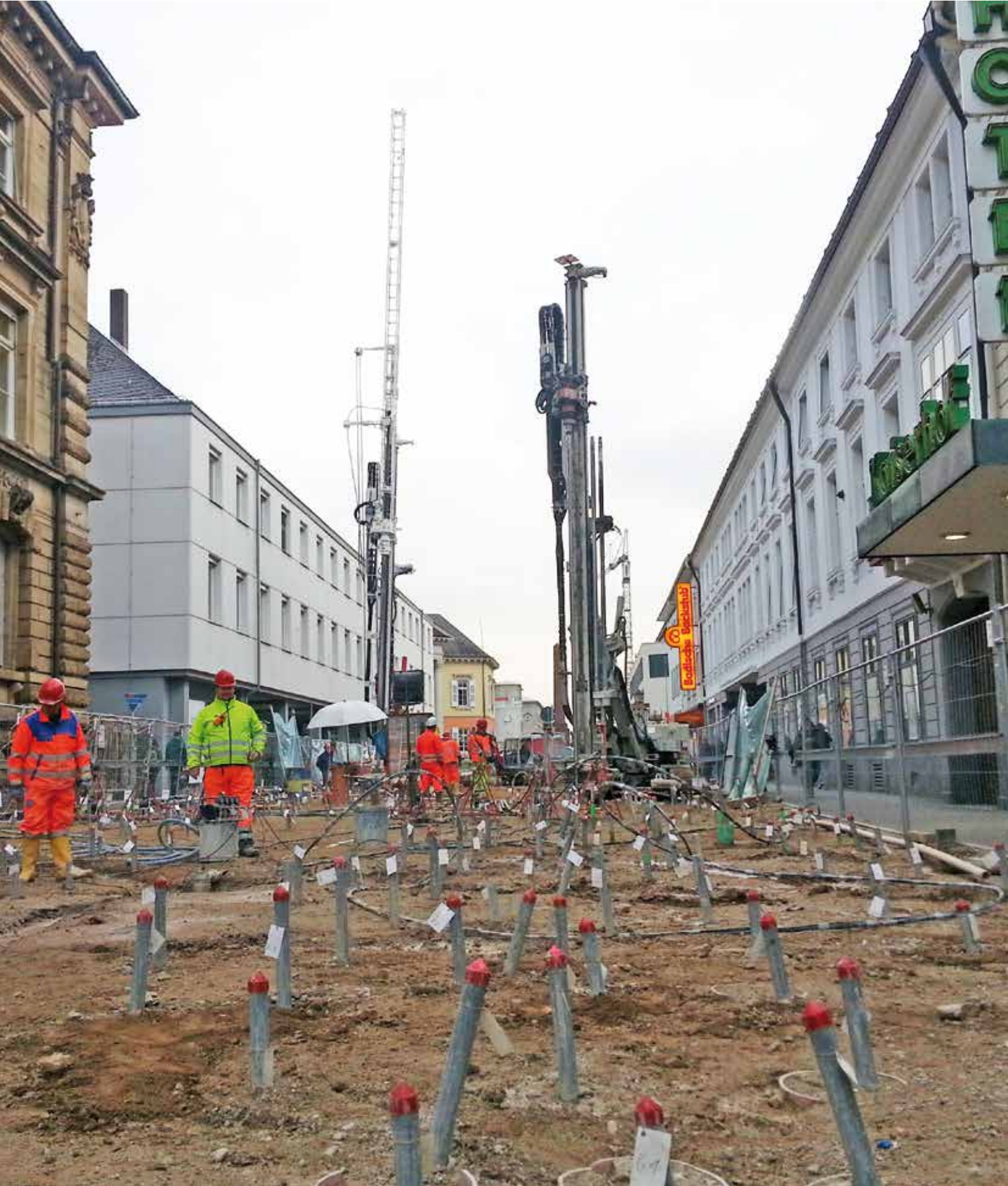
City Metro Tunnel Karlsruhe Manchette Pipe Grouting, Germany Grouting
