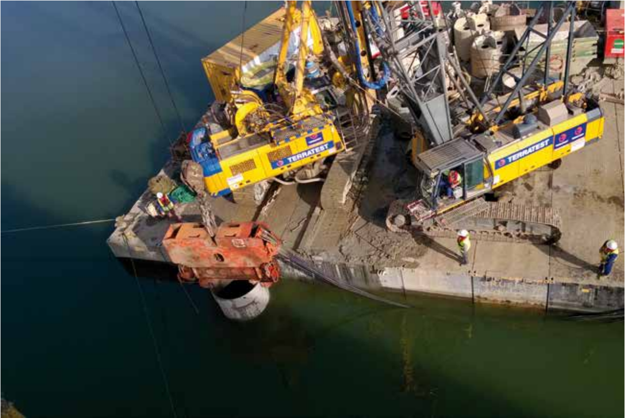
Castiblanco Bridge, Badajoz, Spain Bored Piles
