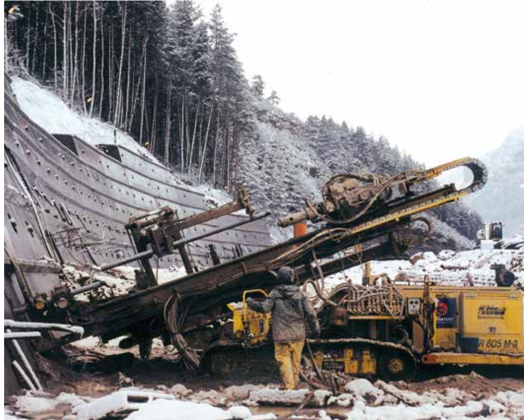
Somport Tunnel. Huesca, Spain Ground Anchors
