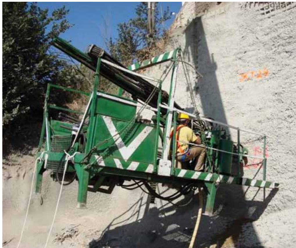
Landslide in Bonares. Huelva, Spain Soil Nailing
