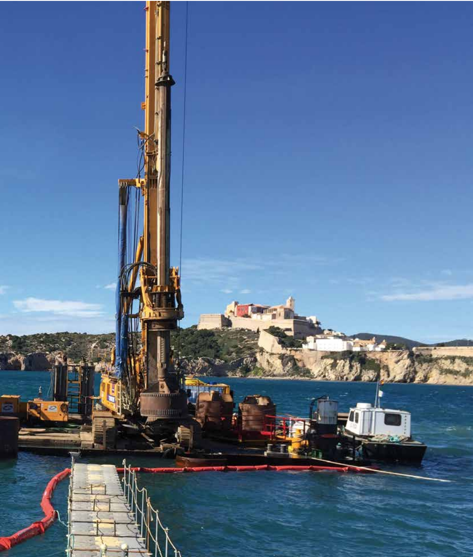
First docking frontline prolongation for large ships. Botafoc Dock. Ibiza, Spain Bored Piles
