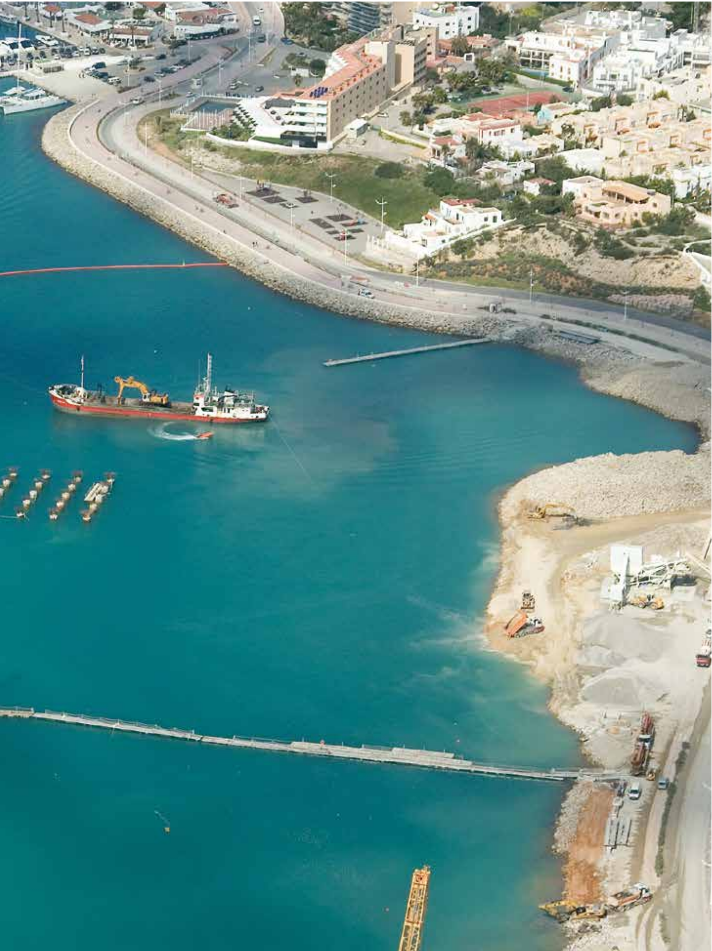
Botafoc Pier. Ibiza Port, Spain Bored Piles
