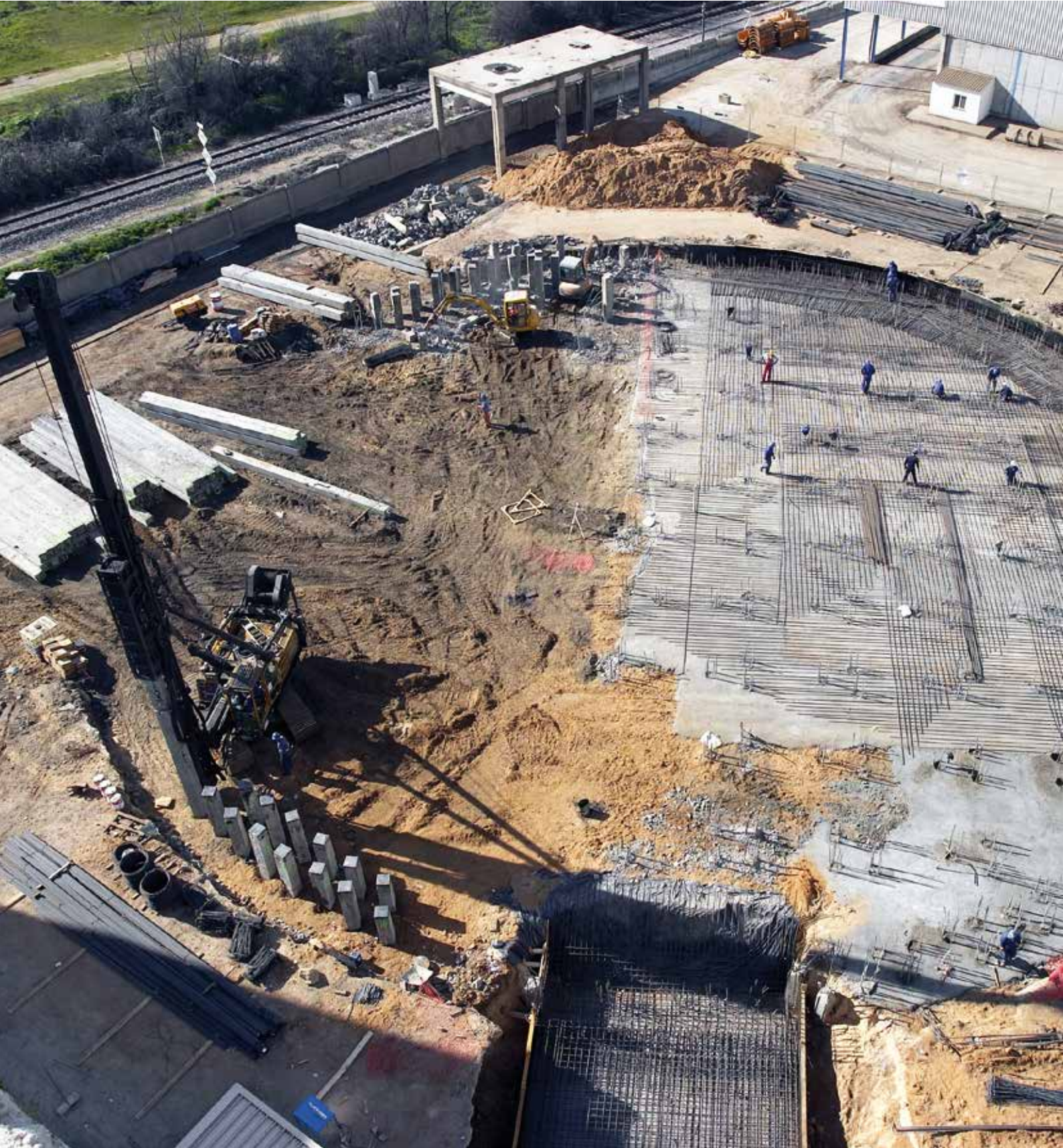
Sugar Silo, Zamora, Spain Precast Piles
