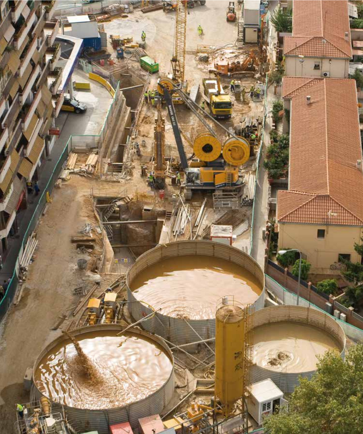
Barcelona Subway, Line 9. Barcelona, Spain Trench cutter
