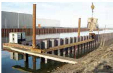
Sheetpiles / Metallic Bracing
