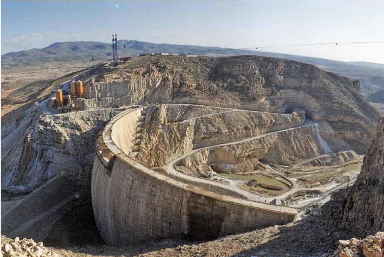
Grass Dam Taourirt Oujda, Morocco Client: KINGDOM OF MOROCCO. MINISTRY OF WORKS Grouting
