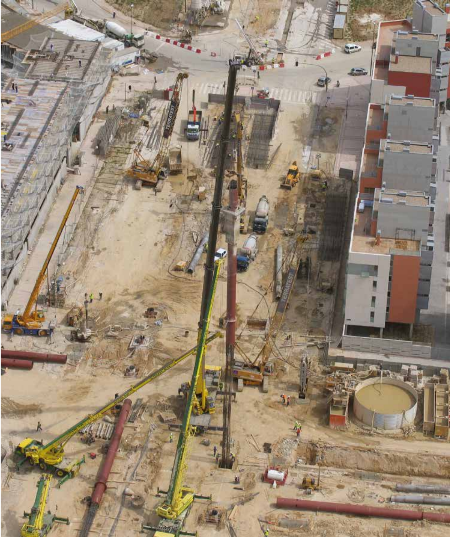
North Subway, Stretch 1A. Madrid, Spain Bored Piles and Diaphragm walls
