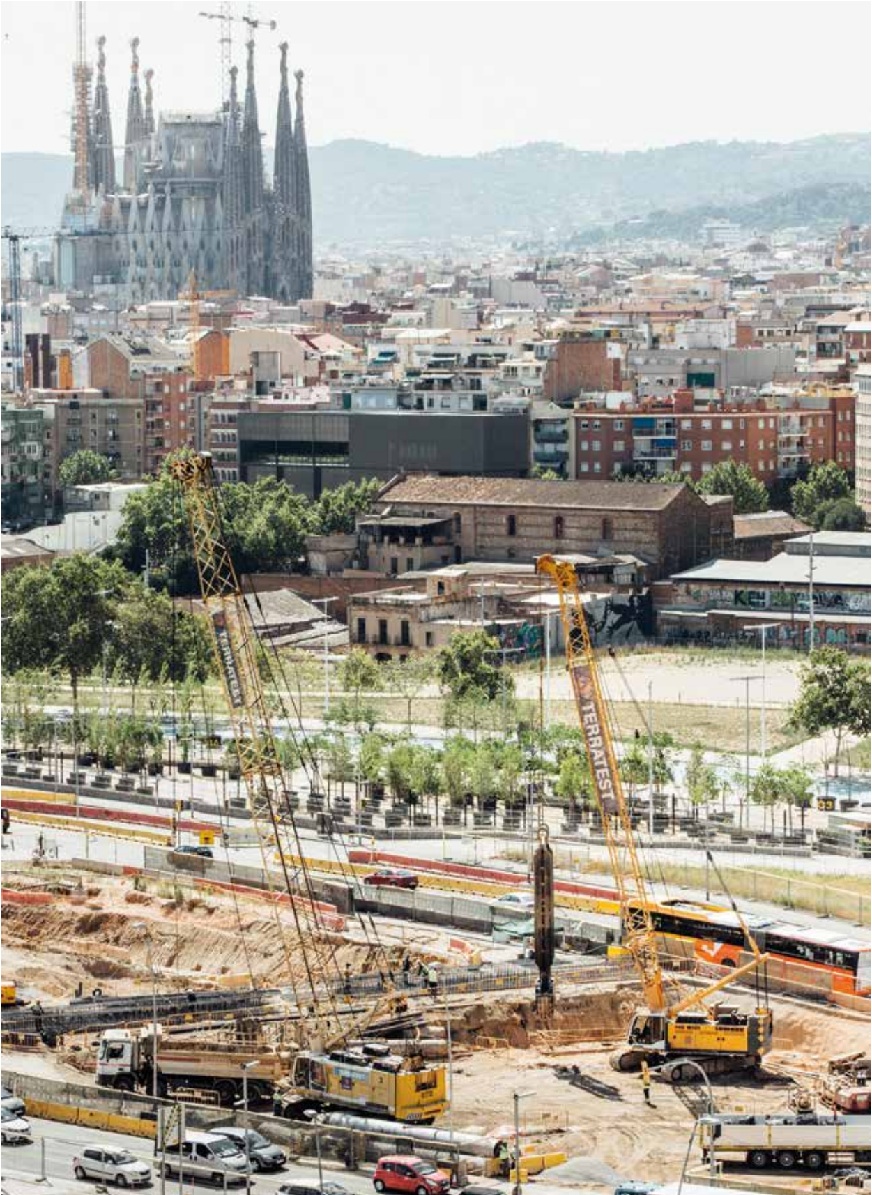
Underpass in the Plaza de les Glòries, Barcelona, Spain Client: UTE Tunel les Glories Diaphragm Walls
