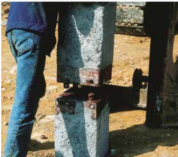
Phase 1: Placing the pile for joining
