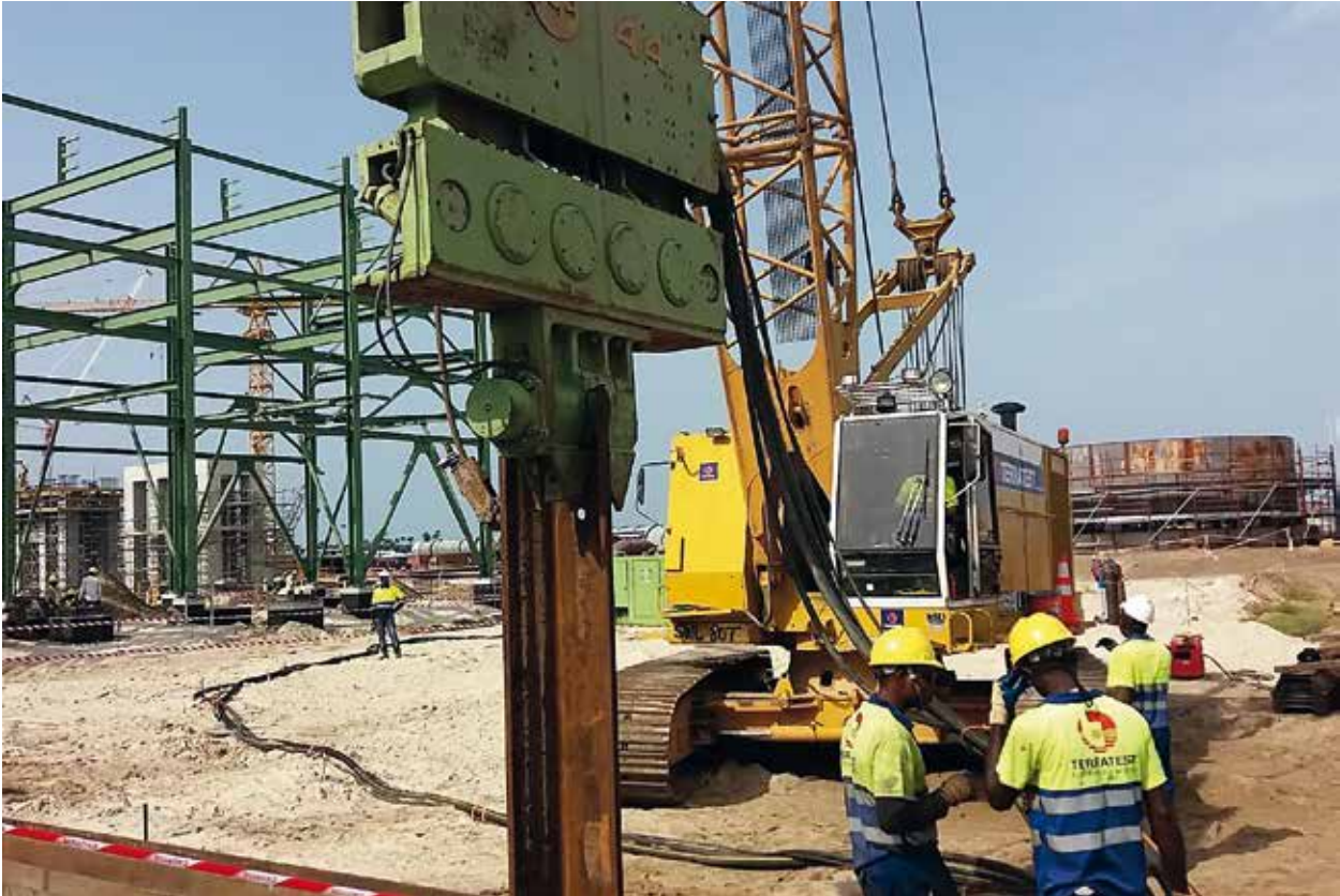
Dangote Fertilizer Plant, Nigeria Client: DANTATA & SAWOE Sheetpiles
