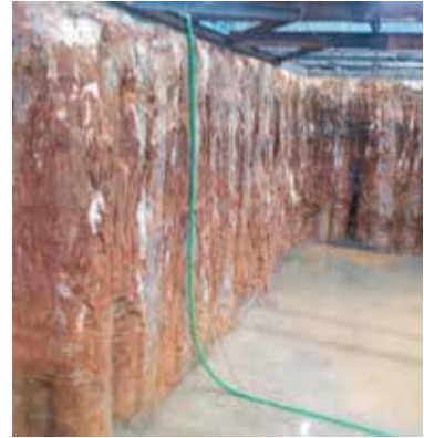
Retaining Wall in Wempeco Factory, Lagos, Nigeria Client: WEMPCO STEEL MILL LIMITED Bored piles
