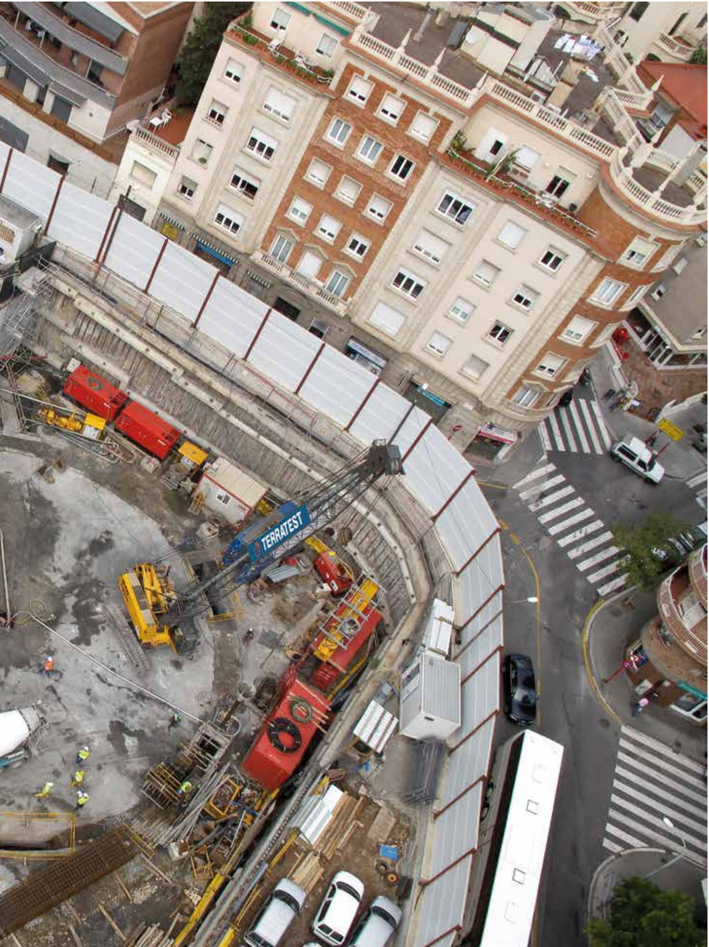
Barcelona Subway, Line 9. Plaza Sanllehy, Barcelona, Spain Trench Cutter
