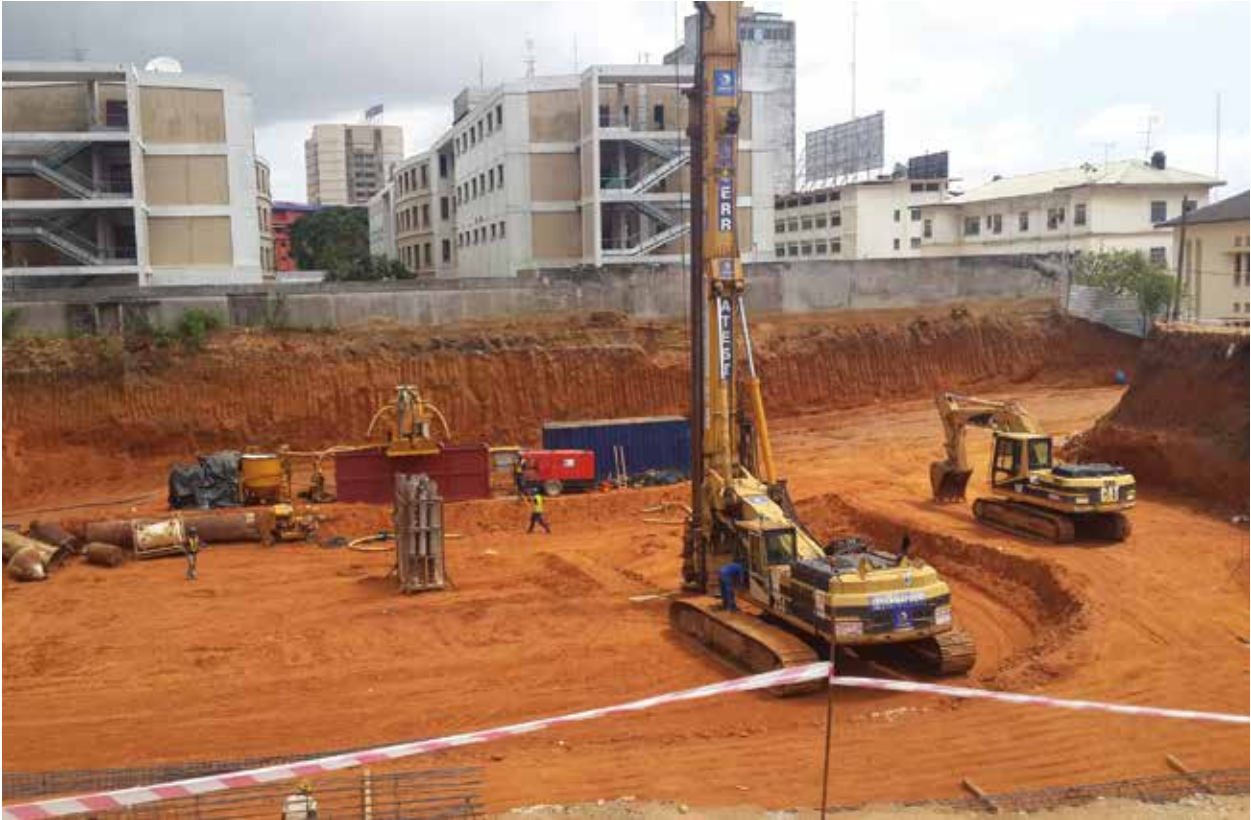
Burkina Faso Embassy in Abidjan, Ivory Coast Client: DECOTEK Bored piles
