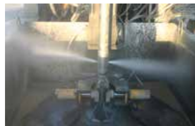
Compensation and Compaction Grouting
