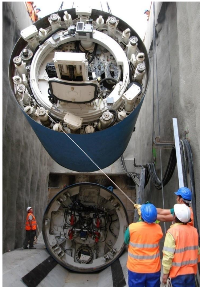
Assembling an EPB machine in the launching shaft
