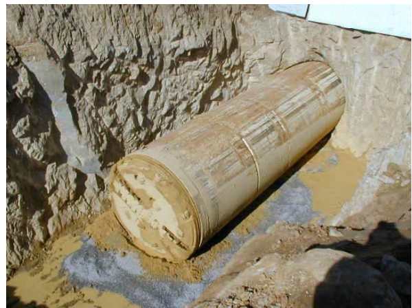
Breakthrough of Hydro shield in reception shaft
