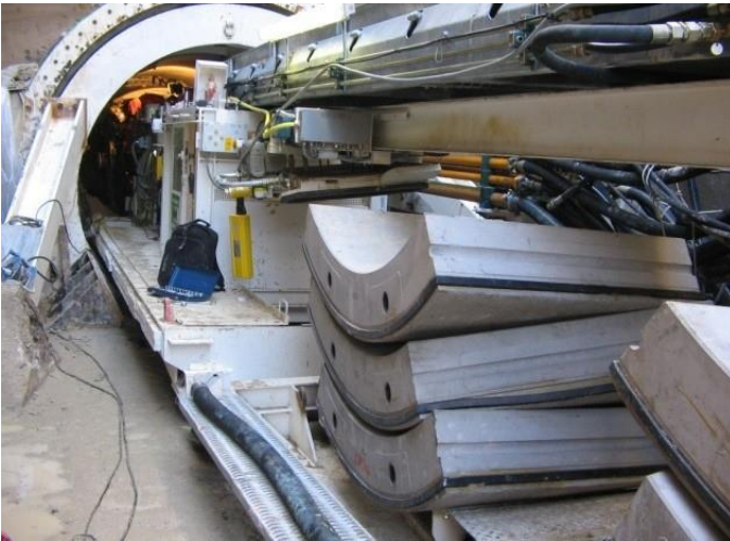
Segments in the Back up of the T.B.M.
