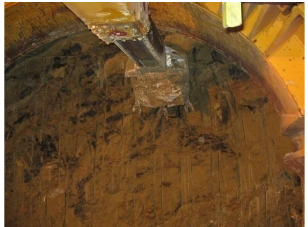
Front face in an excavator open shield
