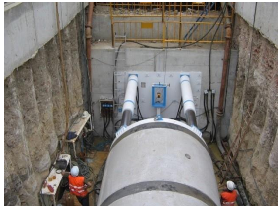
Jacking frame in launching Shaft
