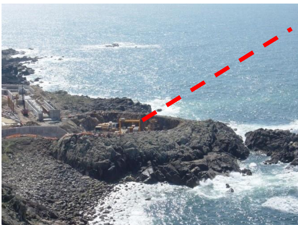
Launch shaft in pipe jacking outfall. A Coruña
