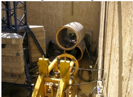
Downloading a jacking pipe
