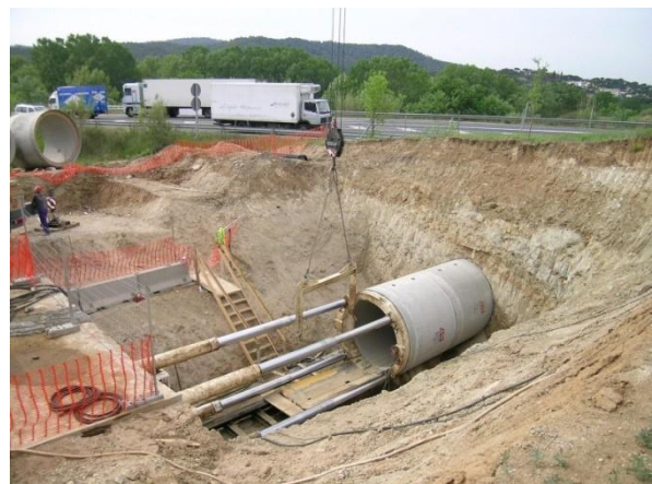
Road crossing with pipe jacking
