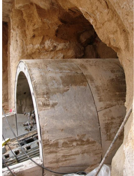
Last lining ring in the reception shaft
