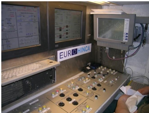
EPB control panel
